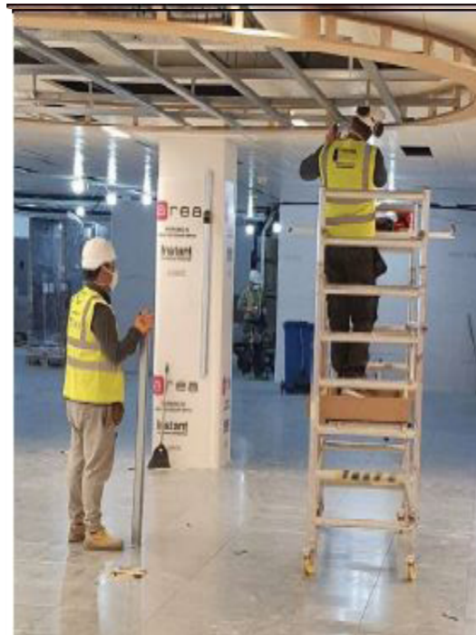
Trade personnel to keep 2m spacing while carrying out works,
